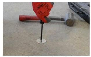
Figure 5. Tightening the Secured Cover
